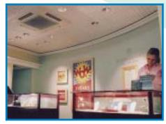
A Chester jewellers has become the first site in the UK to benefit from the new Mitsubishi Electric R410A inverter driven heat pump able to replace old R22 systems using the existing uncleaned pipework.
